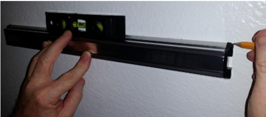
If you are installing into a wall stud behind the dry wall, you will NOT need Wall Anchors; you can drill the screw directly into the wall.
