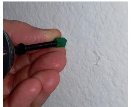
**IMPORTANT:** MAKE SURE the End Cap is aligned to the marking you created above and then drill the screw the remaining way into the wall. Make sure the End Cap is secure into the wall before installing the Magnetic Organizer.
